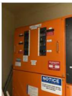
Figure 44: Existing Main Switchboard is to be replaced, with no spatial modifications proposed.
